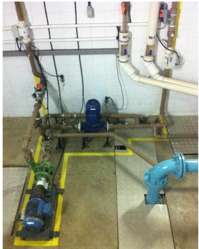
**Fig. 2** Experimental setup 2 – Automated Water Distribution System.
